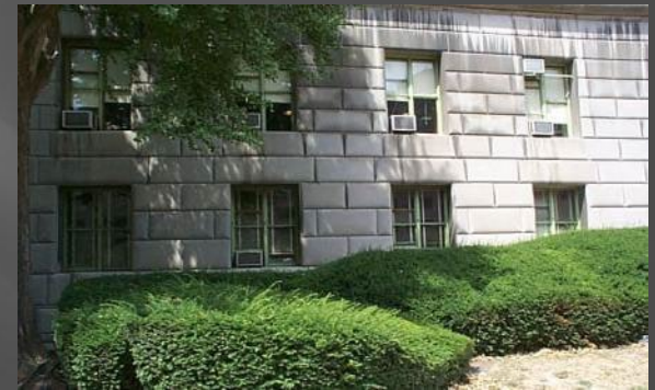
Southern Elevation East Wing Forum Building
