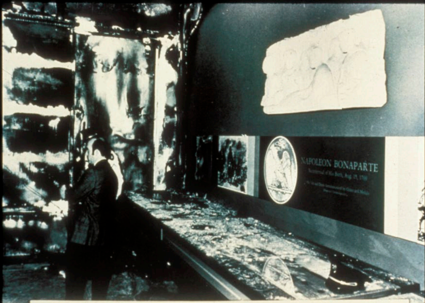
# 6 View of fire damage in the numismatics Hall, looking toward one of the computer exhibit hall doors. Despite the burn-off of combustible
